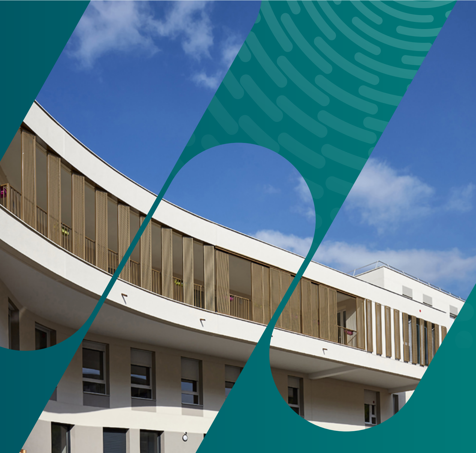
Picture above-Centre Hospitalier de Condrieu - Construction: VINCI - Laboratory equipment: NUVIA
